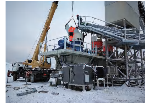
Installation and Commissioning
